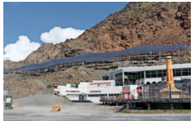
The Pitztaler Gletscherbahnen company has installed a photovoltaic system in the open terrain above the top station of the Gletscherexpress . Commissioned in 2022, it generates almost 1,400 MWh of electricity per year.
