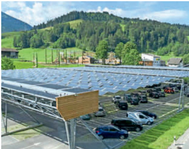
Solar folding roof built over a car park in the Appenzell region. On an area of approx. 4,000 sq.m. the PV system delivers 420 kWp of electricity.
