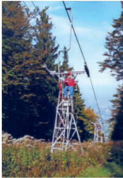
The upper section of the line is flanked by trees.
