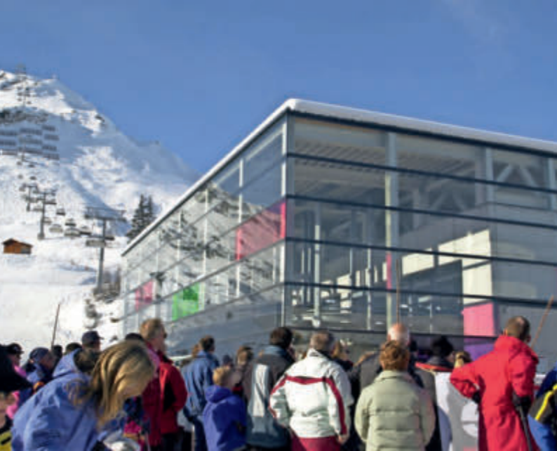
The new bottom station built in 2002 for the Kriegerhorn Cable Car was designed with a façade of photovoltaic panels.
