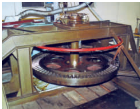
Power transmission from the gearbox to the bullwheel is via an open gearwheel and ring gear.
