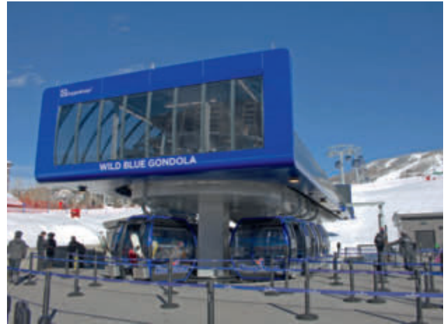
The Wild Blue Gondola is impressive in many ways, e.g. for the world's largest Doppelmayr Direct Drive motor and a line length of over 5 km.
