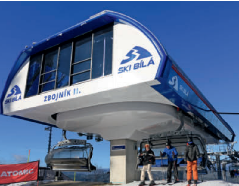
Top station of the new Bílá – Zbojník II 6-seater chairlift
