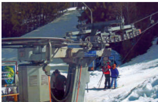
The first Doppelmayr installation on the line of today's chairlift was this surface lift, which is still in operation as a parallel system to the chairlift.
