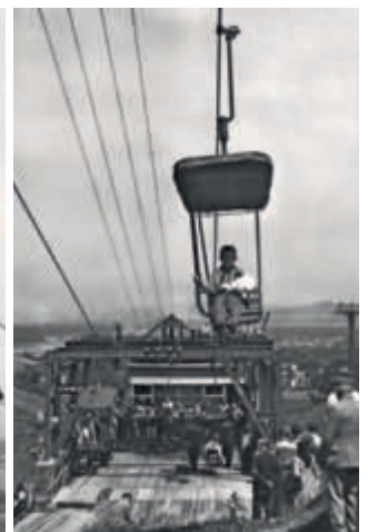
Bottom station in the first years of operation. The station was not originally enclosed; the station building was a later addition.
