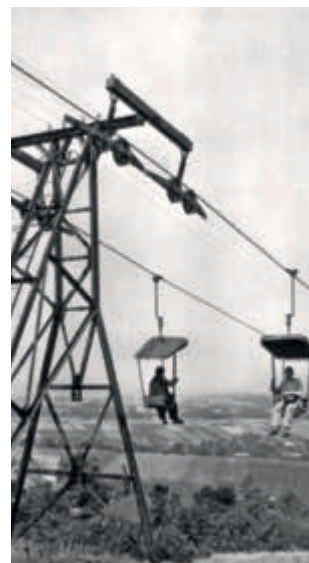
The suspended rope sheaves and the canvas canopy
