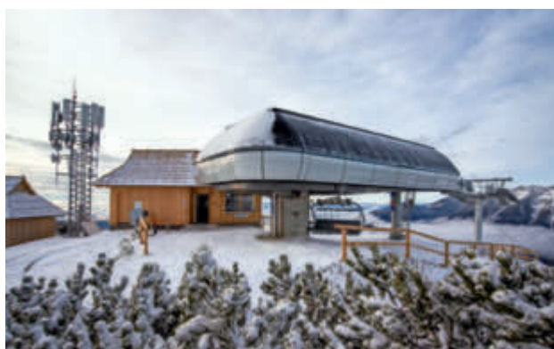
Top station of the CD6 Šimnovec 6-seater chairlift in Velika Planina (SLO) on the 1,666 m high summit of Gradišče
