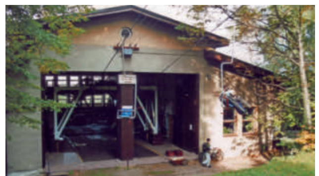
The station building added later
