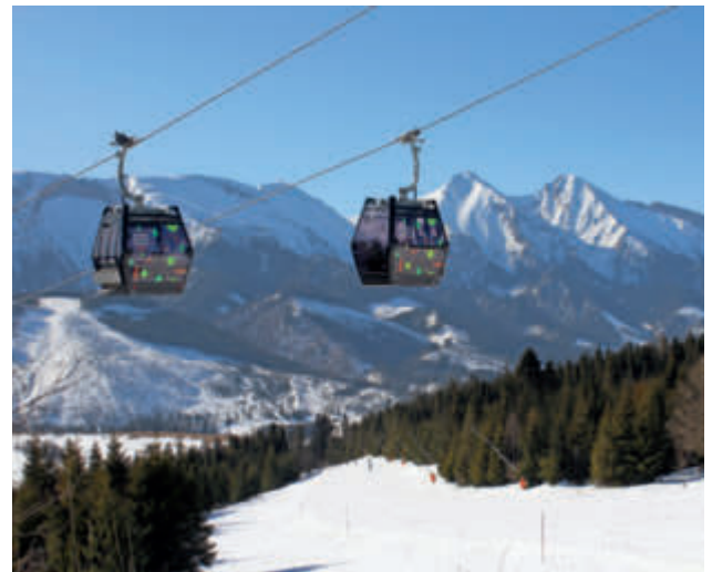
In the Bachledka Ski and Sun resort (SK), where Leitner is building a new 6-seater chairlift this year, this 10-seater gondola lift was opened in 2018.
