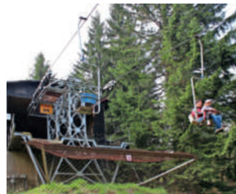
The short pressure frame on the approach to the top station
