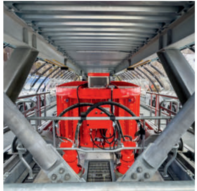
The Leitner DirectDrive in Pamporovo has a rated output of 794 kW.
