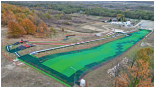
The Neveplast artificial ski slope at the Aprilia Park is 311 meters long.
