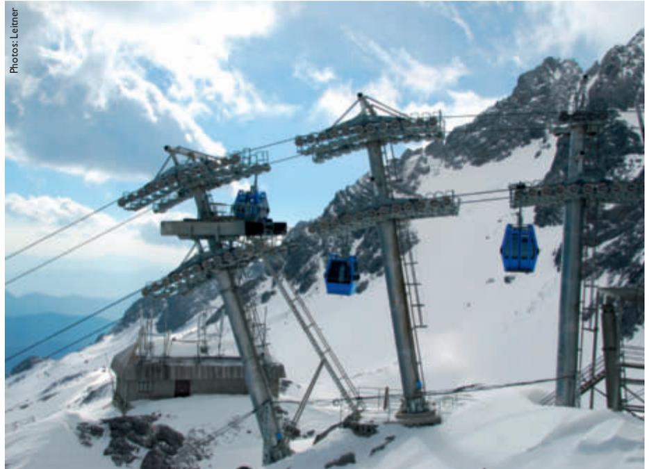
The three-piece tower before the upper terminal is required to handle the evacuation ropeway, with one of the two 6-passenger reversible evacuation cars parked on the lower tower.
