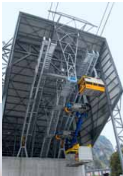
Bottom station of the first stage of Garaventa's heavy-duty ropeway on the construction site of the Limmern power plant
