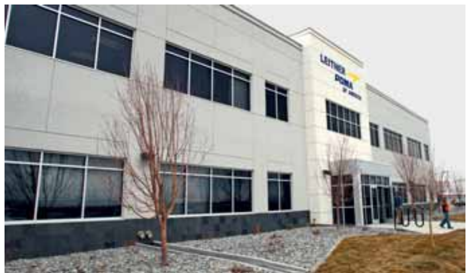
The new Leitner Technologies headquarters in the USA
