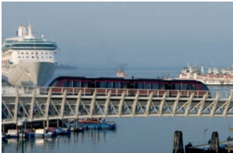
One of the two trainsets on the elevated guideway (Photo: Doppelmayr)
