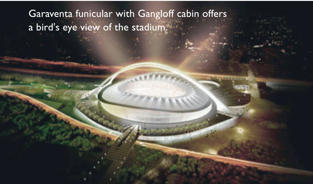
The Garaventa funicular is integrated in the supporting arch of Durban's new Moses Mabhida Stadium.
